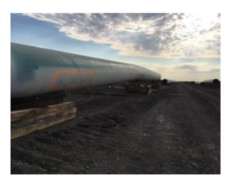
(Left) is a picture of equipment digging ditch.(Right) is a picture of Pipe beside the ditch waiting to be welded together and to be lowered into the ditch.
